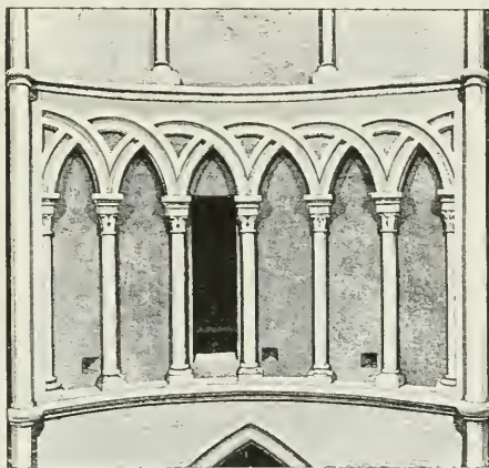
18. Interlacing arcading Triforium, Temple Church.
